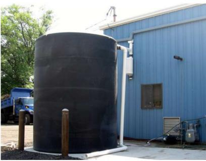
Figure 8a: Rain barrel used to disconnect a downspout with the overflow going to a flower bed
