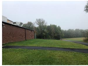
A bioretention system can be installed west of the building to capture, treat, and infiltrate stormwater runoff from the rooftop. A preliminary soil assessment suggests that more soil testing would be required before determining the soil's suitability for green infrastructure.
