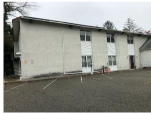
Parking spaces in the parking lot to the west of the building can be converted to porous pavement to capture and infiltrate stormwater runoff from the parking lot. A bioretention system can be installed southeast of the building to capture, treat, and infiltrate stormwater runoff from the roof. A preliminary soil assessment suggests that more soil testing would be required before determining the soil's suitability for green infrastructure.
