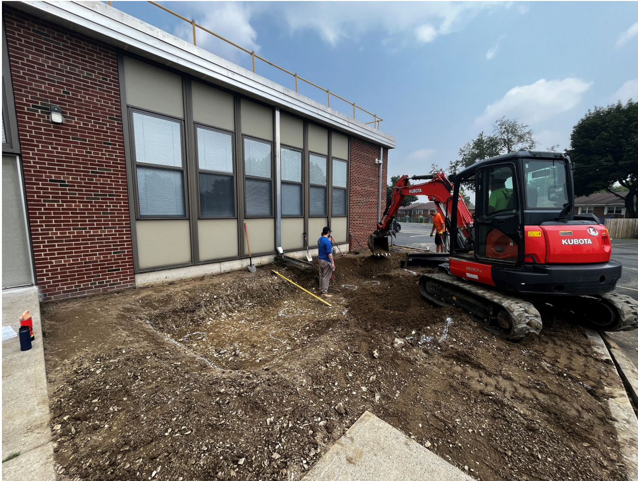
Contractor excavating the rain garden.
