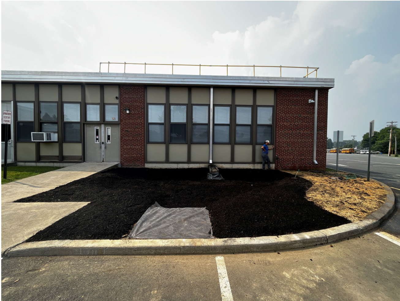
Rain garden following the excavation and mulching.
