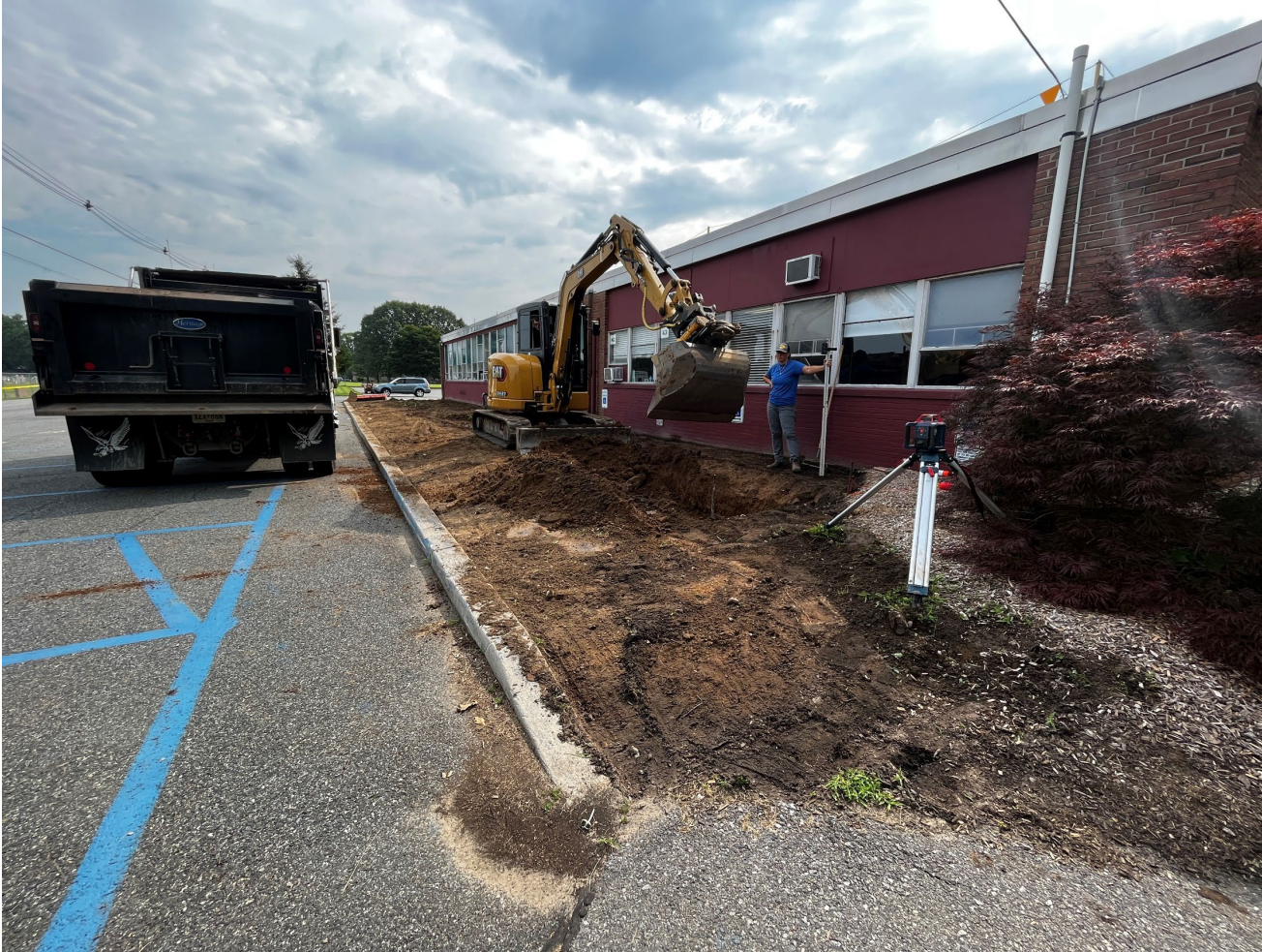
Contractor excavating the rain garden.
