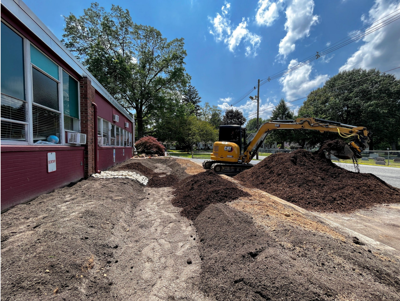
Contractor placing materials in the rain garden.
