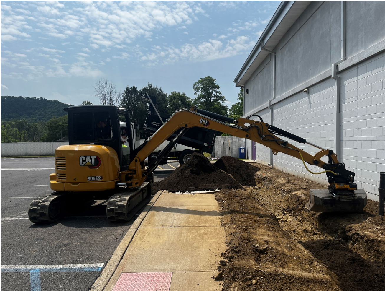
Contractor placing materials in the rain garden.
