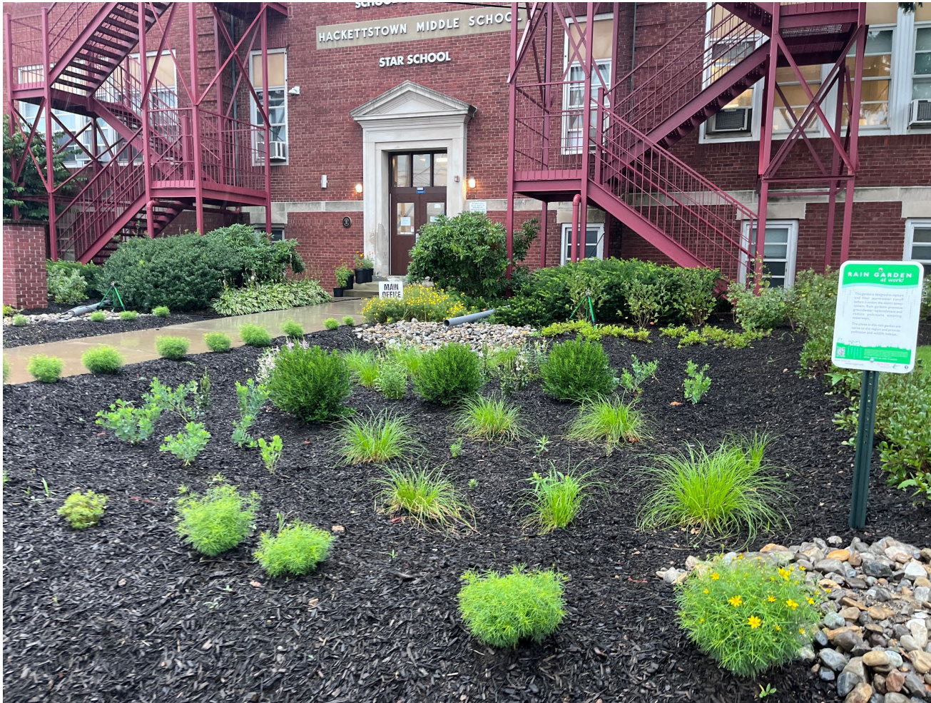
Completed rain gardens.
