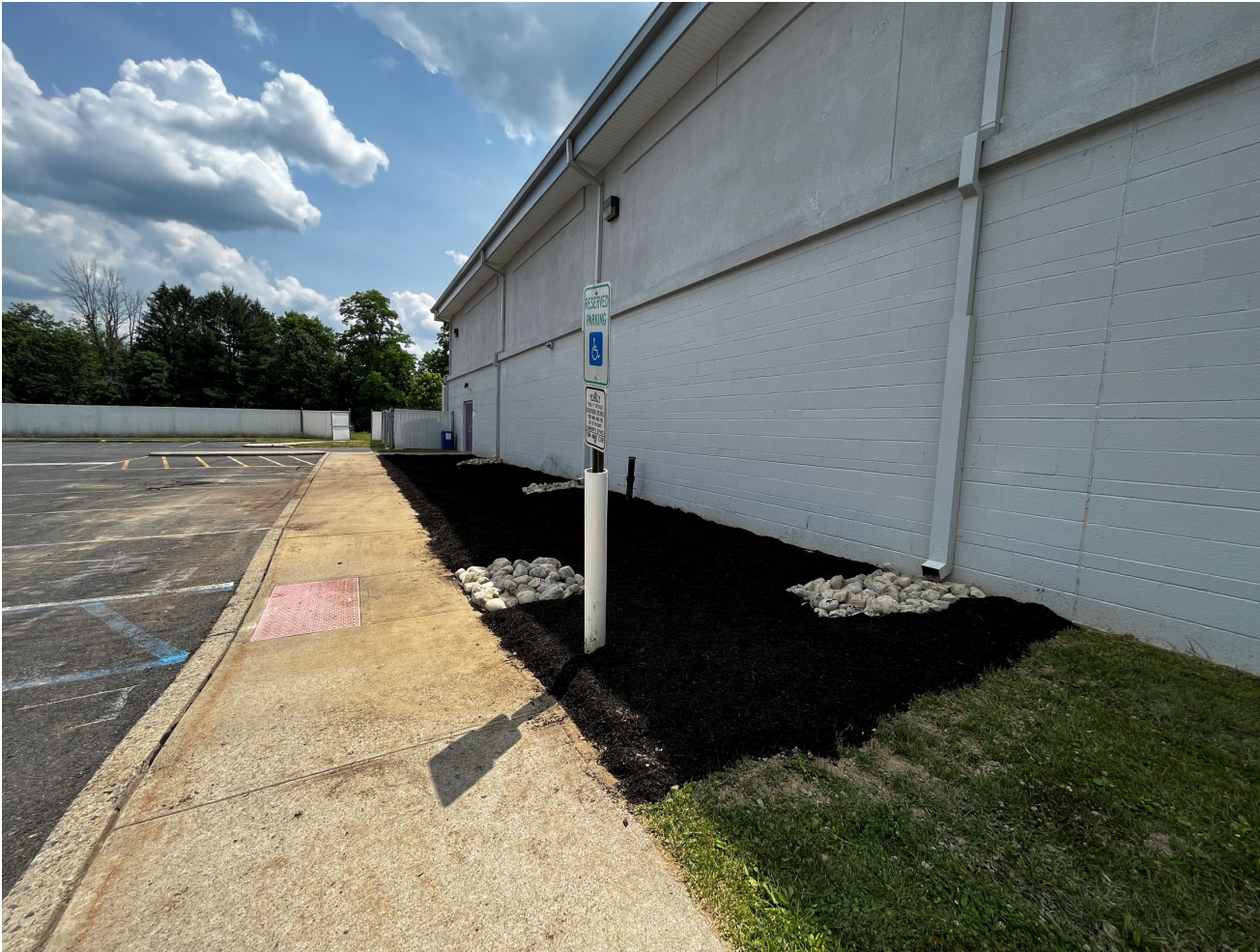
Rain garden following construction.
