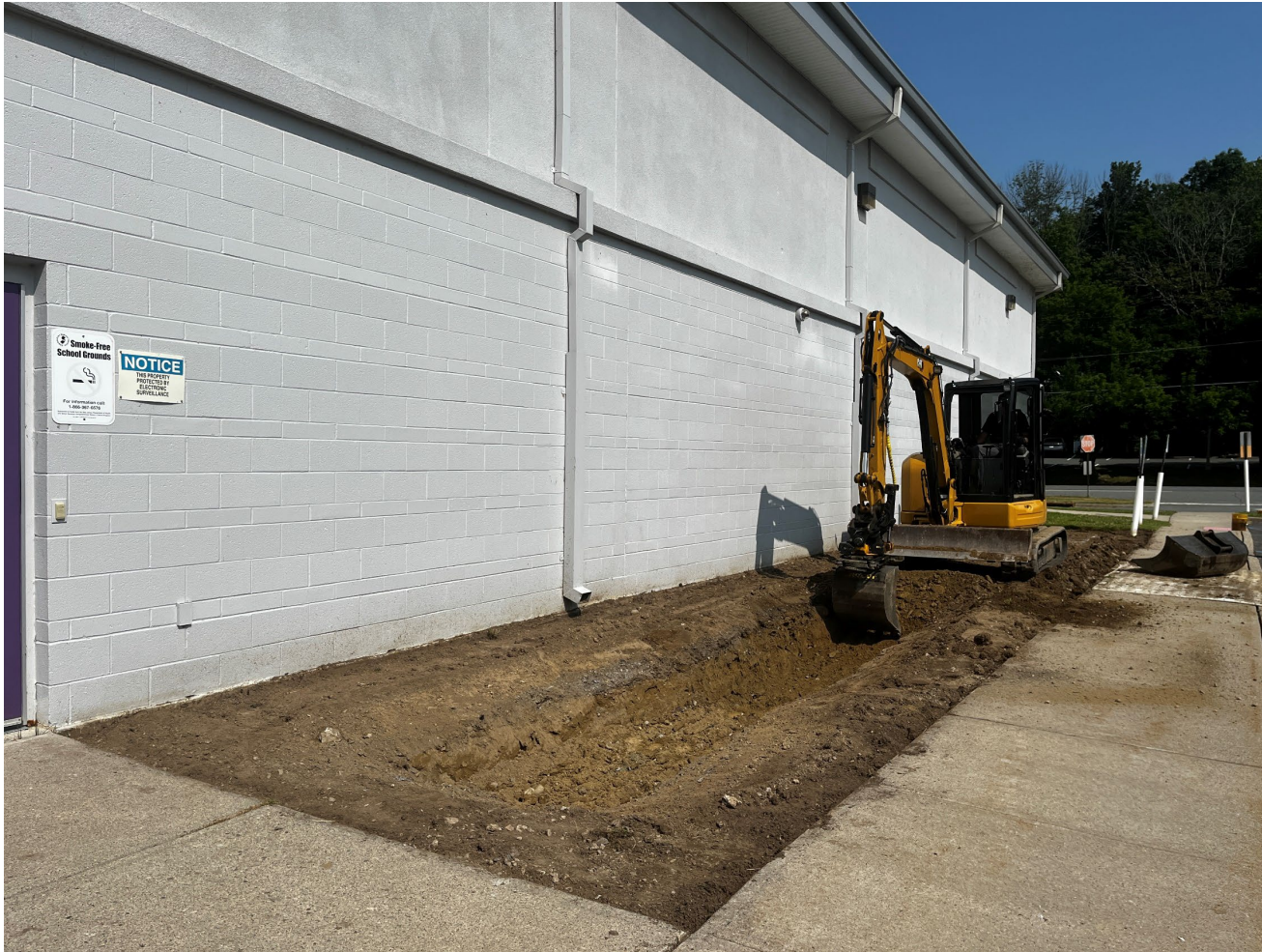
Contractor excavating the rain garden.
