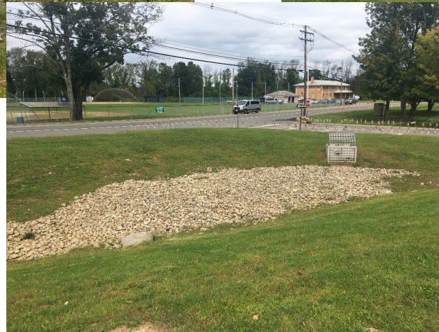
Detention basins prior to project implementation.
