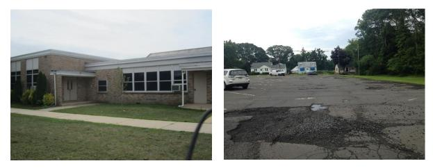
At the time of the assessment, the pavement throughout the school property was in deteriorating condition. Parking spaces can be replaced with pervious pavement to capture and infiltrate stormwater. The rear parking lot is receiving runoff from the roof in addition to the pavement. Installing pervious pavement can capture and infiltrate runoff. A preliminary soil assessment suggests that the soils have suitable drainage characteristics for green infrastructure.
