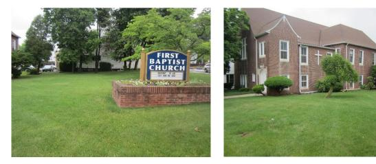
Stormwater planters can be built alongside the street to infiltrate runoff. Downspouts on the northern side of the building can be disconnected into rainwater harvesting systems. A preliminary soil assessment suggests that the soils have suitable drainage characteristics for green infrastructure.
