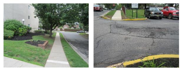
Parking spaces next to the building can be repaved with porous asphalt to infiltrate runoff. A preliminary soil assessment suggests that the soils have suitable drainage characteristics for green infrastructure.
