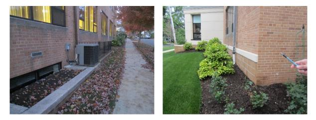
A downspout can be disconnected and directed into a bioretention system near the corner of 3rd Avenue and Summit Place, which will capture, treat and infiltrate roof runoff. A preliminary soil assessment suggests that more soil testing would be required before determining the soil's suitability for green infrastructure.
