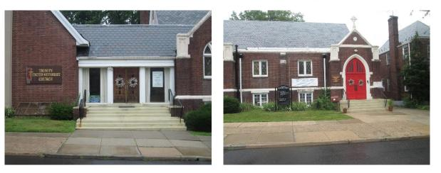
Two downspouts on the western side of the building can be disconnected into rainwater harvesting systems. The driveway on the eastern side of the building can be repaved with porous asphalt in order to infiltrate roof runoff. A preliminary soil assessment suggests that soils have suitable drainage characteristics for green infrastructure.
