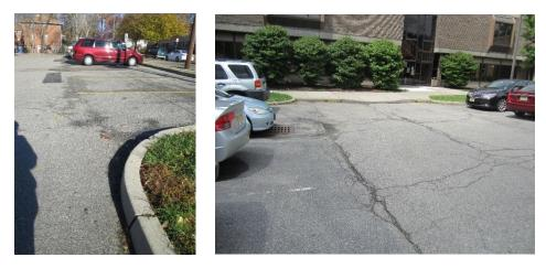
Parking spaces and a portion of the sidewalk can be repaved with porous pavements to infiltrate stormwater. A rain garden can also be installed to capture, treat, and infiltrate runoff. A preliminary soil assessment suggests that the soils have suitable drainage characteristics for green infrastructure.
