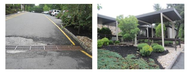
A portion of the drive lane near the River Road entrance can be replaced with porous pavement to capture stormwater from the parking lot. On the eastern side of the building, a downspout can be disconnected into a rainwater harvesting system. A preliminary soil assessment suggests that the soils have suitable drainage characteristics for green infrastructure.
