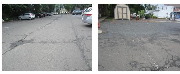
A portion of the parking lot can be repaved with porous asphalt to manage stormwater. The optimal locations for this porous asphalt would be uphill of three existing catch basins. A preliminary soil assessment suggests that the soils have suitable drainage characteristics for green infrastructure.
