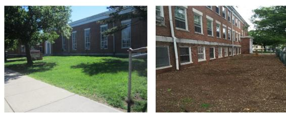
Two bioretention systems can be installed to capture, treat, and infiltrate rooftop runoff by disconnecting and redirecting downspouts into them. A preliminary soil assessment suggests that more soil testing would be required before determining the soil's suitability for green infrastructure.
