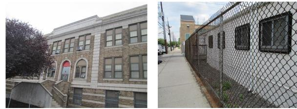
Almost all of the elementary school is made up of impervious cover, including asphalt in front of the entrance. This area can be depaved and converted into rain gardens to capture, treat and infiltrate runoff. A preliminary soil assessment suggests that more soil testing would be required before determining the soil's suitability for green infrastructure.
