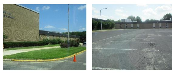
Stormwater is currently directed to an existing detention basin. Parking spots can be replaced with porous asphalt to capture and infiltrate stormwater. A preliminary soil assessment suggests that more soil testing would be required before determining the soil's suitability for green infrastructure.
