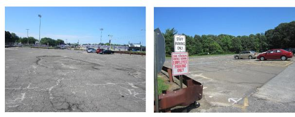
Parking spaces north of the school and near the baseball field can be replaced with porous asphalt to capture and infiltrate stormwater. A preliminary soil assessment suggests that the soils have suitable drainage characteristics for green infrastructure.
