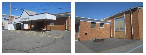
Parking spaces around the school can be replaced with porous asphalt to capture and infiltrate stormwater. A preliminary soil assessment suggests that the soils have suitable drainage characteristics for green infrastructure.
