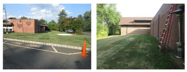
Parking spaces can be replaced with pervious pavement to capture and infiltrate runoff. Bioretention systems can be installed to capture, treat, and infiltrate rooftop runoff. A preliminary soil assessment suggests that the soils have suitable drainage characteristics for green infrastructure.
