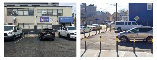
Eastern parking spaces in the parking lot can be converted to porous pavement to capture and infiltrate stormwater runoff from the parking lot. A preliminary soil assessment suggests that more soil testing would be required before determining the soil's suitability for green infrastructure.
