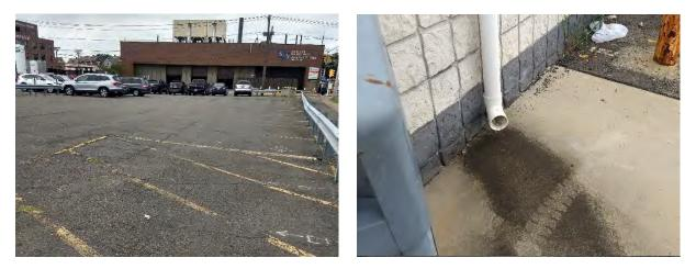
The southern parking spaces can be converted to pervious pavement to capture and infiltrate the stormwater runoff from both the rooftop and parking lot. A preliminary soil assessment suggests that more soil testing would be required before determining the soil's suitability for green infrastructure.
