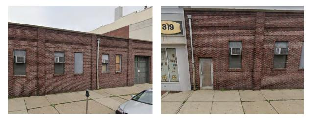
Downspout planter boxes can be installed on the northern side of the building to treat the stormwater runoff from the rooftop. A preliminary soil assessment suggests that more soil testing would be required before determining the soil's suitability for green infrastructure.
