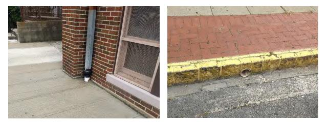
Downspout planter boxes can be installed south of the building on the connected downspouts to treat the stormwater from the rooftop before it is discharged to the street. A preliminary soil assessment suggests that more soil testing would be required before determining the soil's suitability for green infrastructure.
