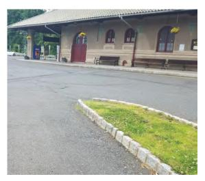
Downspouts on the north and south of the building can be disconnected and converted to planter boxes to capture stormwater runoff from the roof. Sections of parking spaces can be converted to porous pavement to capture and infiltrate stormwater runoff from the parking lot. A preliminary soil assessment suggests that more soil testing would be required before determining the soil's suitability for green infrastructure.
