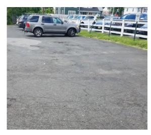
Parking spaces in the parking lot to the north of the building can be converted to porous pavement to capture and infiltrate stormwater runoff from the parking lot. On the north side of the building downspout planter boxes can be installed to help capture stormwater runoff from the building's roof. A preliminary soil assessment suggests that more soil testing would be required before determining the soil's suitability for green infrastructure.
