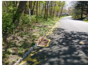
A bioswale can be installed west of the existing catch basin in the grassed area between the tree cover. The catch basin had standing water in it so an investigation to the downhill piping could help with water ponding issues in this area. A preliminary soil assessment suggests that the soils have suitable drainage characteristics for green infrastructure.
