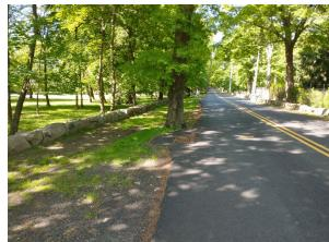
A stone swale can be installed south of Mountain Top Road to help guide the water flow away from the retaining wall toward the catch basin on the corner of the roadway. A bioswale can be installed west of Overleigh Road in the existing eroded area to aid in water conveyance to the nearby catch basins. A preliminary soil assessment suggests that more soil testing would be required before determining the soil's suitability for green infrastructure.
