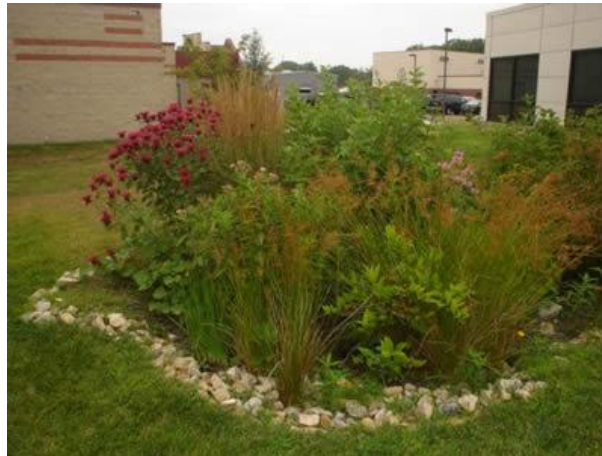
Figure 7: Rain garden outside the RCE of Gloucester County office which was designed to disconnect rooftop runoff from the local storm sewer system
