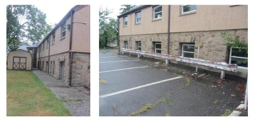
Parking spaces can be replaced with pervious pavement to capture and infiltrate stormwater. Additionally, a rain garden can be installed near the entrance of the building to capture, treat, and infiltrate roof runoff. A preliminary soil assessment suggests that the soils have suitable drainage characteristics for green infrastructure.
