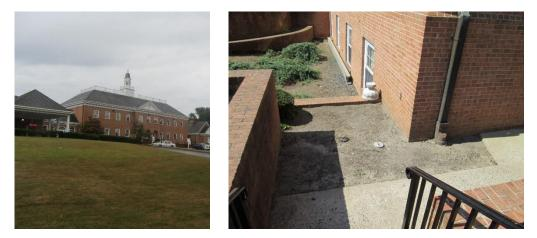
Two downspout planter boxes can be constructed and placed at downspouts to allow roof runoff to be reused. A rain garden can be built in the turf grass south of the building to capture, treat, and infiltrate runoff. parking spots can be replaced with pervious pavement to infiltrate rainwater. A preliminary soil assessment suggests that the soils have suitable drainage characteristics for green infrastructure.
