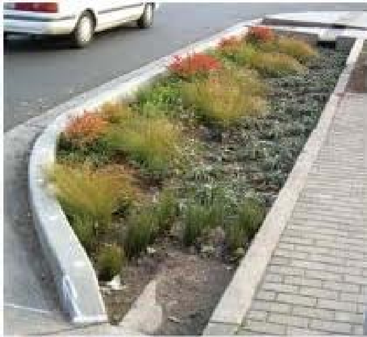
Curb extension with a planted swale that captures stormwater from the gutter. Portland, OR (Credit: Abby Hall)
