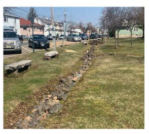
An existing rock swale can be converted to a bioswale to aid in infiltration of the stormwater runoff entering it. Additionally, the parking spaces to the west of the park can be converted to pervious pavement to capture, treat, and infiltrate the stormwater runoff from the parking lot. A preliminary soil assessment suggests that more soil testing would be required before determining the soil's suitability for green infrastructure.
