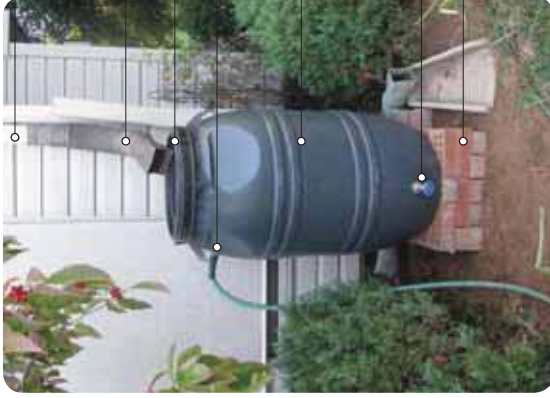
Example of a residential rainwater harvesting system
