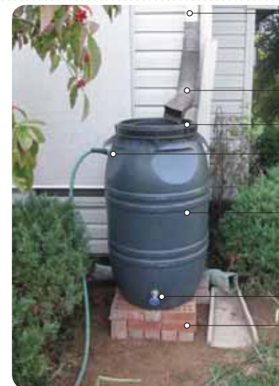
Example of a residential rainwater harvesting system
