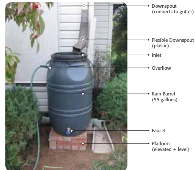
Example of a residential rainwater harvesting system
