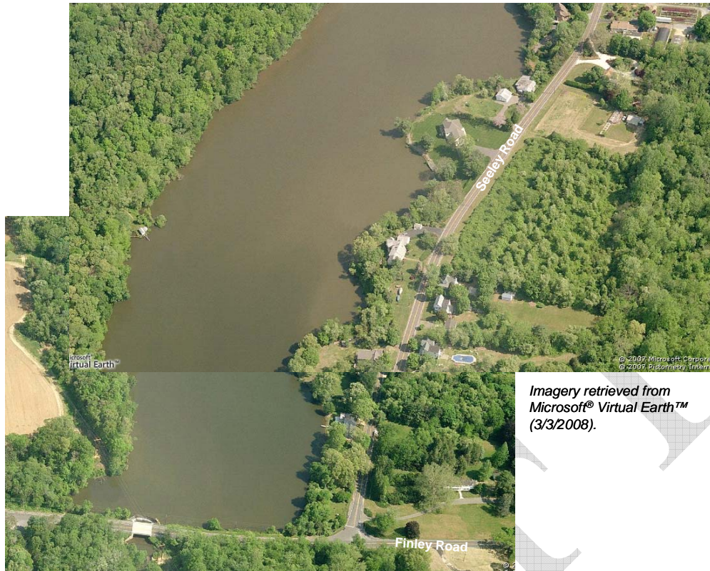
Figure B-4: Seeley Lake and its spillway to the Cohansey River.
