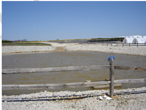
Figure B-8: Basins collect runoff from nursery acreage.
