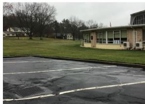
Rain gardens can be installed in the turfgrass areas near the east side entrance of the building to capture, treat, and infiltrate stormwater runoff from the roof. Parking spaces in the parking lot to the north of the building can be converted to pervious pavement to capture and infiltrate stormwater runoff from the pavement. A preliminary soil assessment suggests that more soil testing would be required before determining the soil's suitability for green infrastructure.
