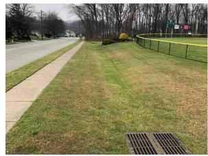
A bioswale can be installed in the turfgrass depressed area near the entrance of the complex to convey, treat, and infiltrate stormwater from the pavement. Pervious pavement can be installed in the parking spaces on the east side of the lot to intercept water before reaching the catch basins. A preliminary soil assessment suggests that more soil testing would be required before determining the soil's suitability for green infrastructure.
