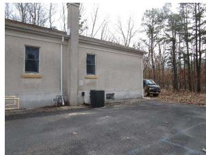
Downspout planter boxes can be constructed along the northwest and southeast sides of the building to allow roof runoff to be reused. A preliminary soil assessment suggests that the soils have suitable drainage characteristics for green infrastructure.
