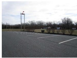
Two rain gardens can be installed at the two north corners of the building to capture, treat, and infiltrate rooftop runoff. The southernmost row of parking spaces can be replaced with pervious pavement to capture and infiltrate stormwater. A preliminary soil assessment suggests that more soil testing would be required before determining the soil's suitability for green infrastructure.
