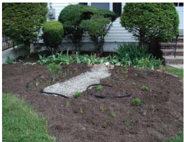
At time of installation Springfield Township Municipal Annex Building Springfield, NJ
