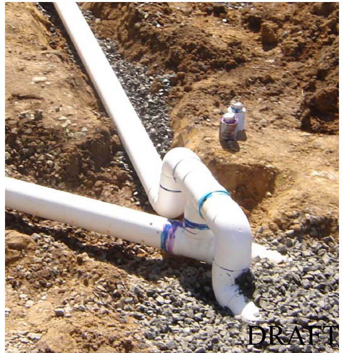
CONNECTION TO EXISTING UNDERDRAIN
