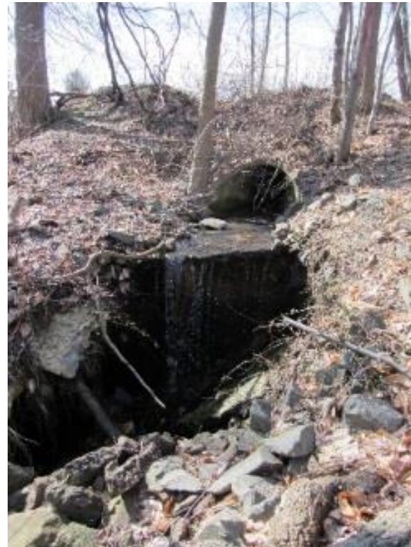
Outlet Destabilization
