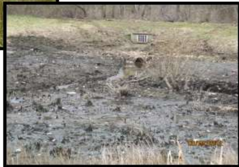
Kristopher Drive Basin After Cleaning (2012)
