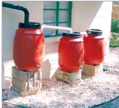
Multiple barrels provide for greater water storage.
