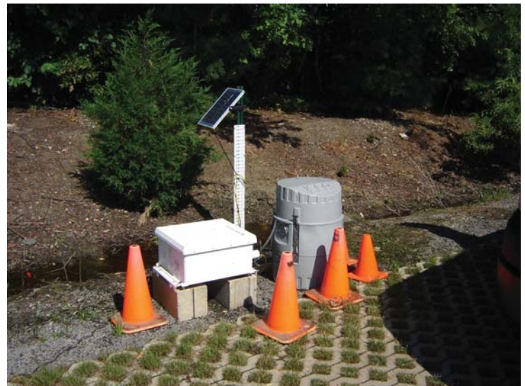
Monitoring station at Pinelands Nursery
