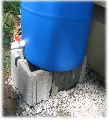
Rain barrel needs to be higher than ground level
