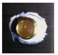
Caulk around inside of overflow fitting
