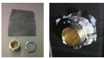
Screw lock nut over screen on the inside of overflow fitting.
