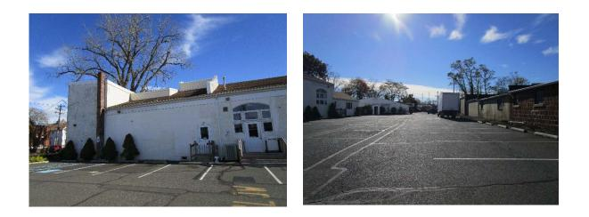
Parking spots can be replaced with porous asphalt to capture and infiltrate stormwater from the parking lot and rooftop by directing downspouts into it. A preliminary soil assessment suggests that the soils have suitable drainage characteristics for green infrastructure.
