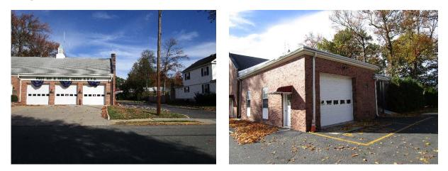
Roof runoff can be harvested by installing a cistern at the northeast corner of the building. The water can then be used for watering gardens, washing vehicles, or for other non-potable uses. Installing a rain garden in front of the building can capture, treat, and infiltrate roof runoff. A preliminary soil assessment suggests that the soils have suitable drainage characteristics for green infrastructure.
