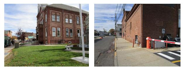
Installing a rain garden adjacent to the building can capture, treat, and infiltrate roof runoff. A stormwater planter can be constructed to the south of the building by directing the downspout that is already routed under the sidewalk into the planter. A preliminary soil assessment suggests that more soil testing would be required before determining the soil's suitability for green infrastructure.
