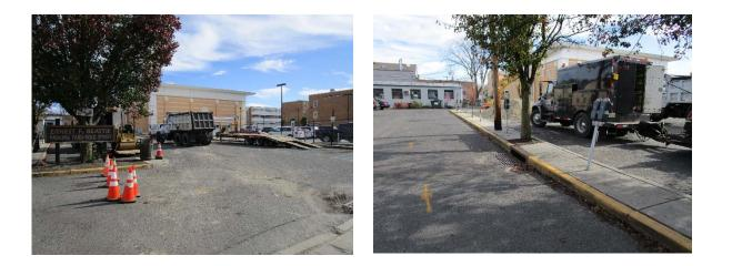
Parking spots along the street can be replaced with porous asphalt to capture and infiltrate stormwater. A preliminary soil assessment suggests that more soil testing would be required before determining the soil's suitability for green infrastructure.
