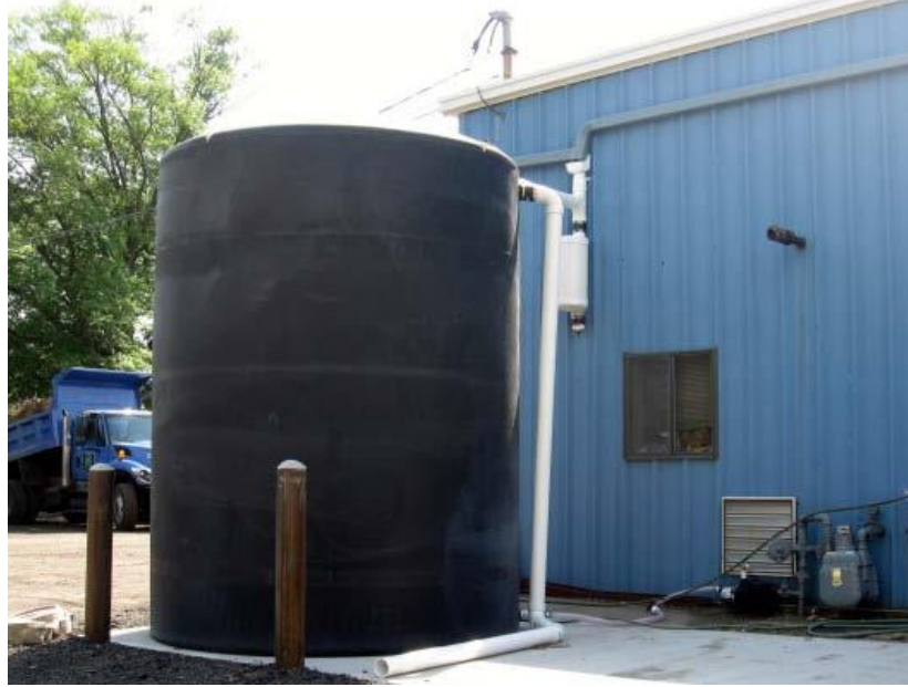
Figure 8b: A 5,000 gallon cistern used to disconnect the rooftop of the Department of Public Works in Clark Township to harvest rainwater for nonprofit car wash events
