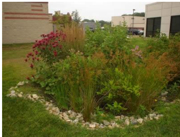
Figure 7: Rain garden outside the RCE of Gloucester County office designed to disconnect rooftop runoff from the local storm sewer system
