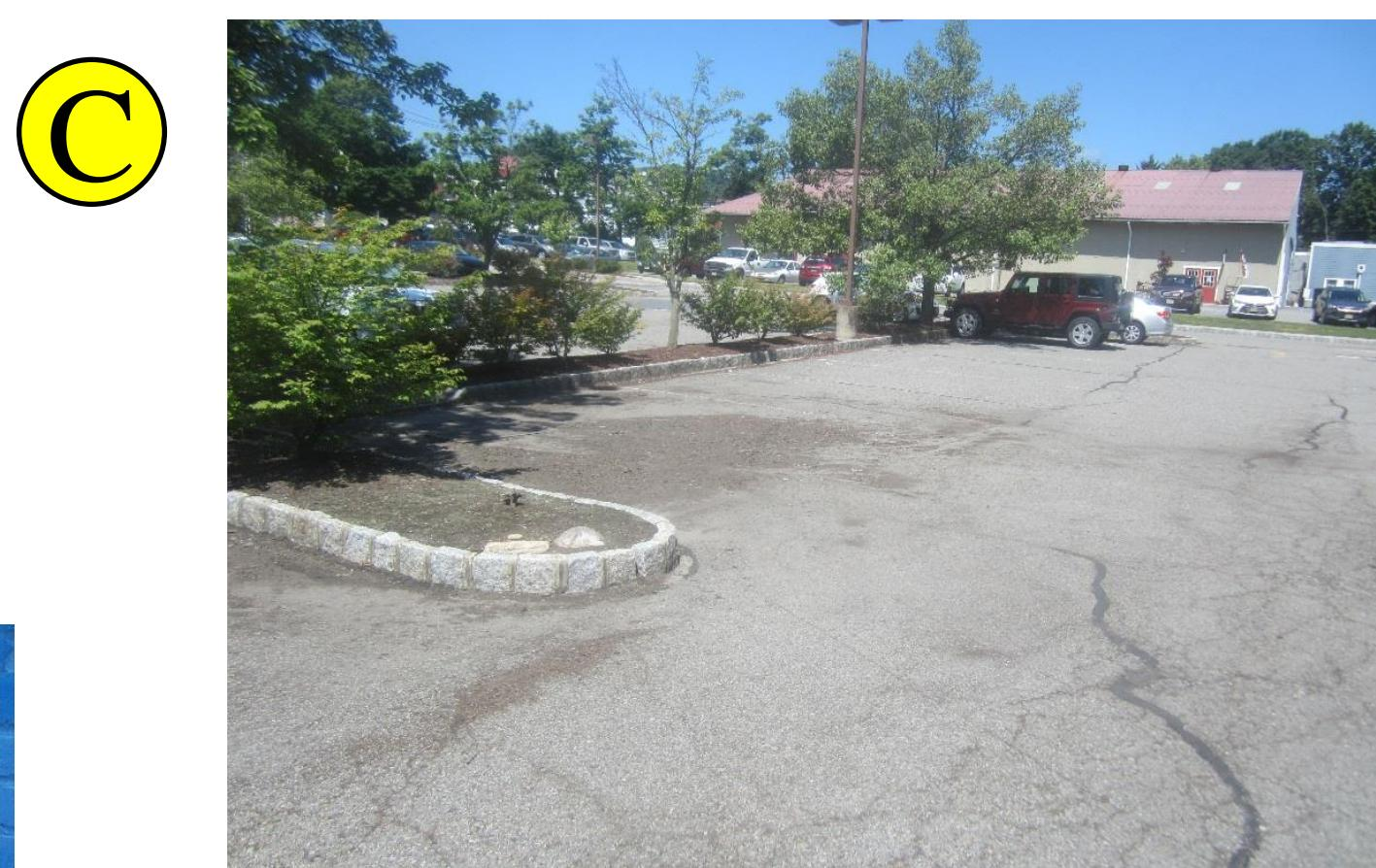
**1 BIORETENTION SYSTEMS:** Rain gardens will be used to reduce sediment and nutrient loading to the local waterway and increase groundwater recharge. This site has four locations for rain gardens: along the northwest side, at the east corner, and at the south corner. All of these rain gardens collect runoff from downspouts.
