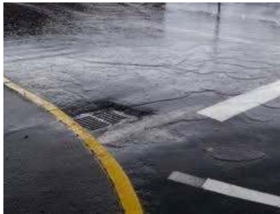
Figure 1: Stormwater draining from a parking lot
